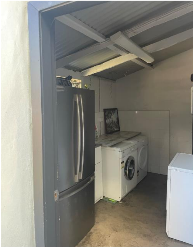
Figure 6: Existing skillion addition comprising laundry which is proposed for demolition
