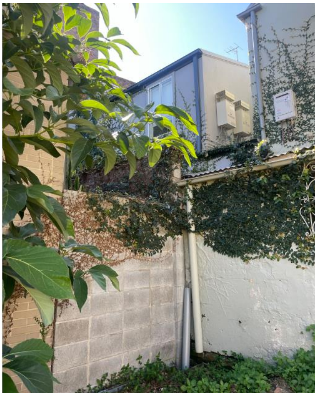
Figure 5: Photograph showing skillion addition (proposed for demolition) abutting adjoining development located at 191 Harris Street
