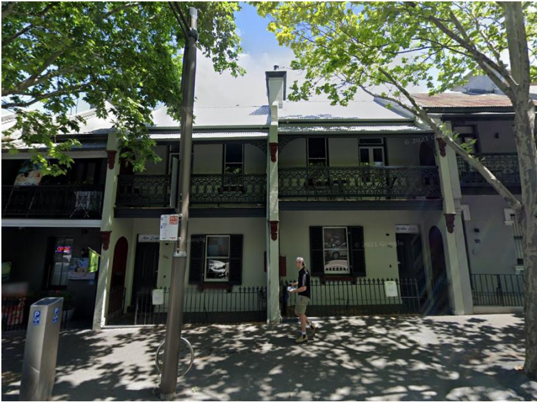
Figure 2: View of terrace from Harris Street, the subject site is the green terrace located on the right-hand side
