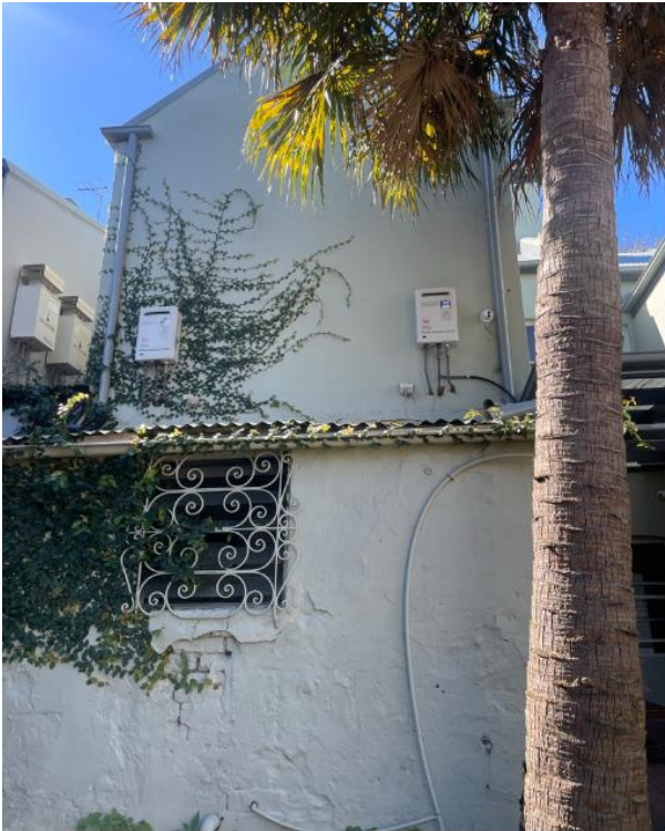
Figure 4: Photograph showing skillion addition to rear which is proposed for demolition and existing cabbage tree palm
