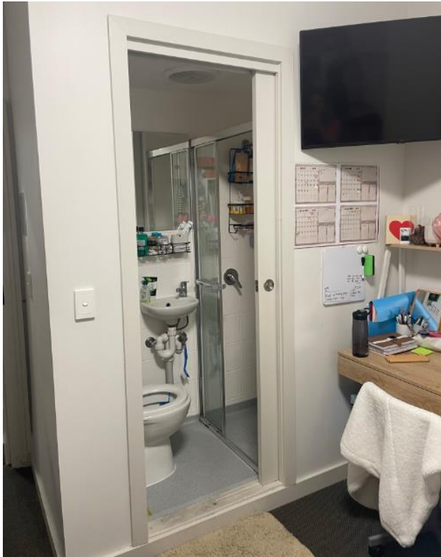
Figure 12: Room 5 with ensuite bathroom constructed without development consent
