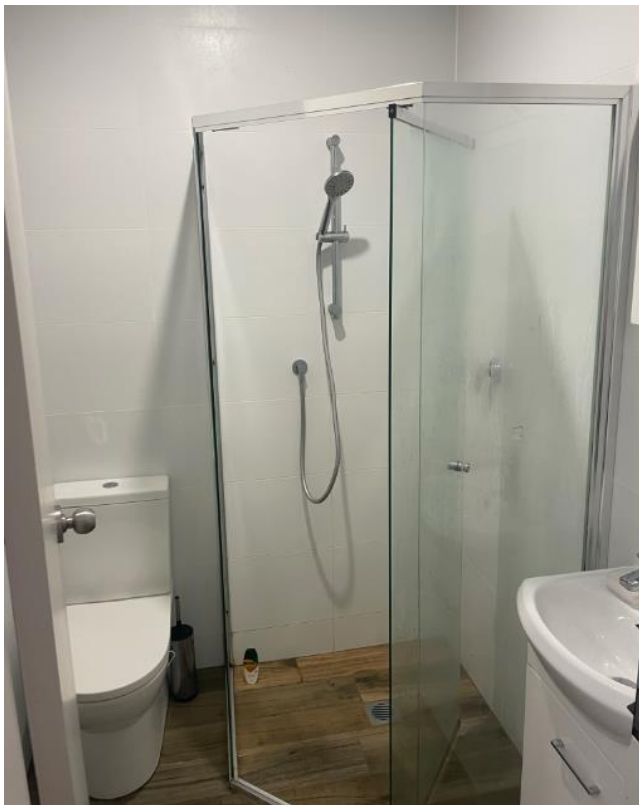
Figure 11: Former kitchen which has been converted into three separate bathrooms without development consent
